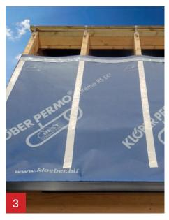
Fix 50mm Butylon® tape down the rafters to seal around any nail penetrations.
