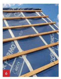
Fix battens and continue process until underlay installation is completed.
