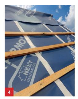
Install battens fixing nails through Butylon® tape and lay next layer of Permo® extreme RS with a 100mm headlap so adhesive strips meet.
