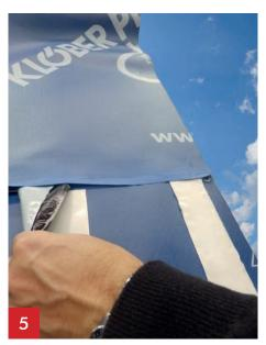
Peel back adhesive tape on the two strips sticking the two together.
