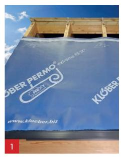
Lay the Permo $^{\text{®}}$  extreme RS with a drape of 10-15mm between the rafters.
